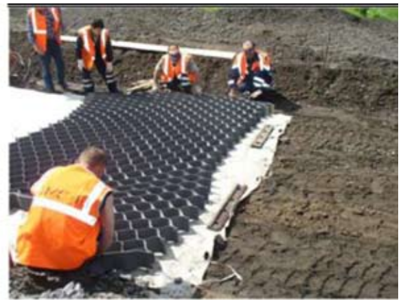
Picture 9 The layering of the protection sub-ballast layer with using of the geocell on the geotextile and sand- gravel mix (Zaytsev A.A., Bubnovsky V.V. 2014)
